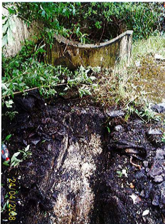
Photograph 11: Photograph showing location of TP4, within southern section of the site. Blackened near surface materials visible in foreground and concrete supports for AST visible in background.
