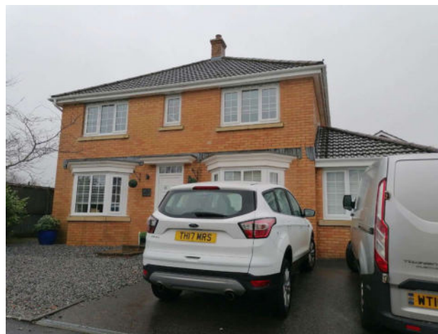
Dwellings adjacent to site in Crymlyn Gardens
