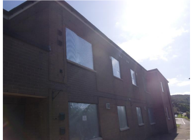
Figure 8 - Western aspect of the building
