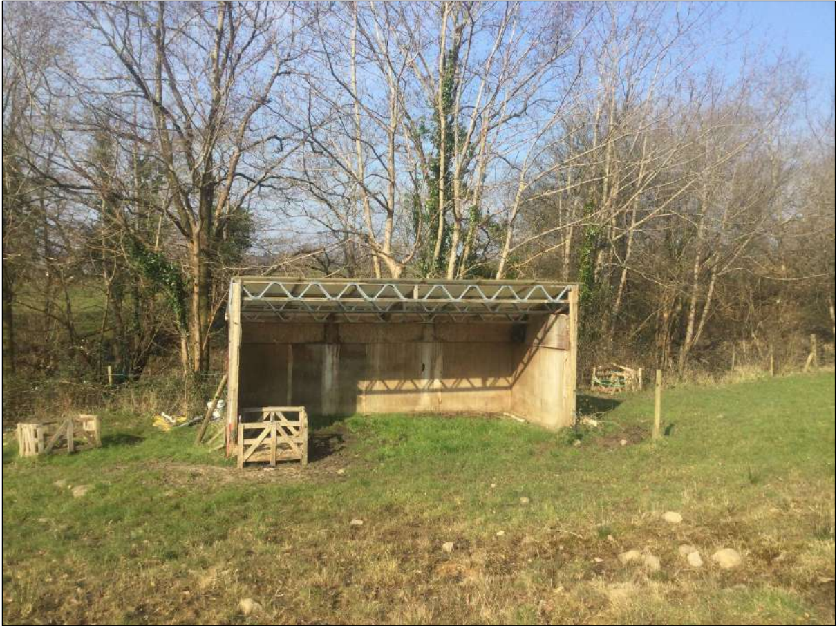
Plate 9. Prefabricated livestock shed within the application area.
