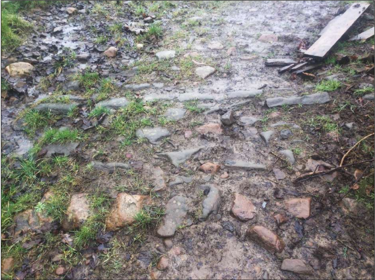
Plate 19. Remains of a cobbled metalled surface running north-west/south-east into Sites northern boundary.
