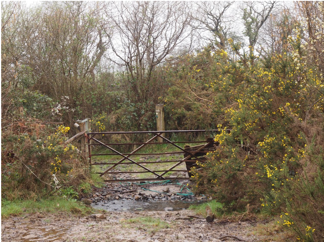
Image EDP 4.1: Site access gates in poor condition along western boundary.
