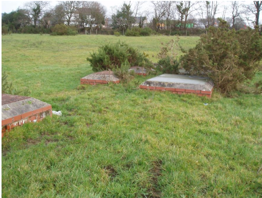
Evidence of construction drainage works (TN2).
