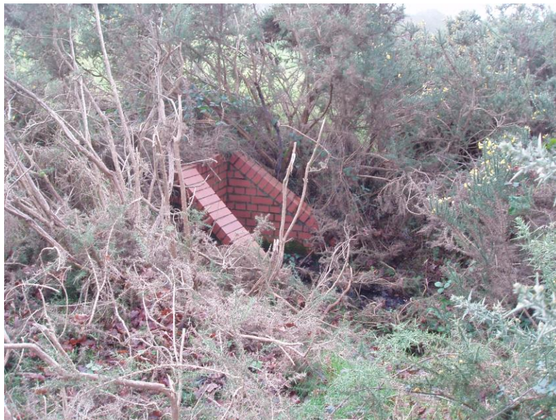
Culvert exit, TN8
