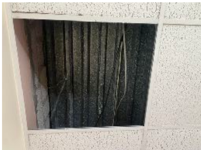
Example View of internal roof view
