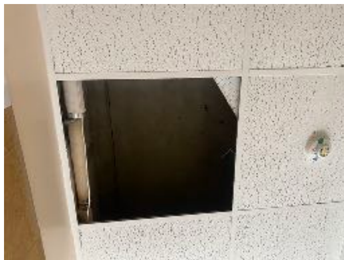
Example View of internal roof view
