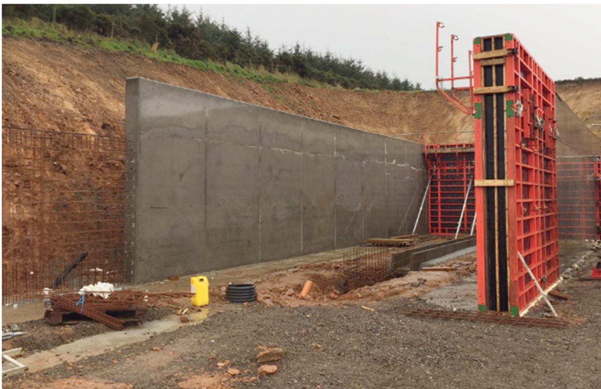
Figure 6: Concrete retaining walls construction sequencing
