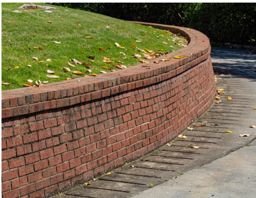
Figure 3: Picture of brick retaining wall
