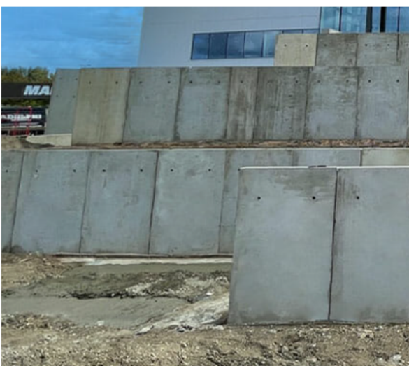
Figure 5: Precast concrete retaining walls
