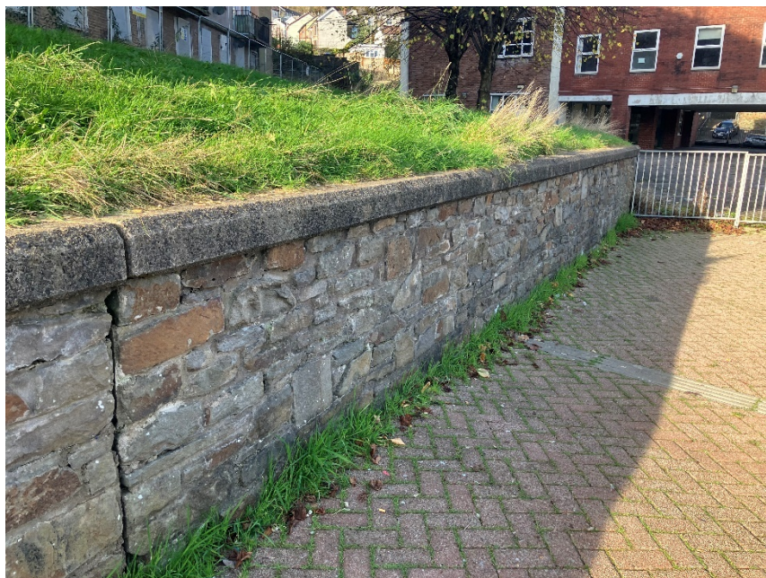
Figure 13: Stone wall located on site boundary
