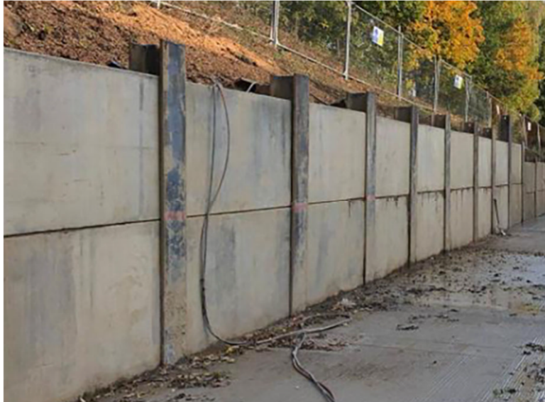
Figure 7: King-post retaining wall
