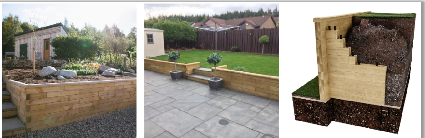
Figure 1: Low height timber retaining structures
