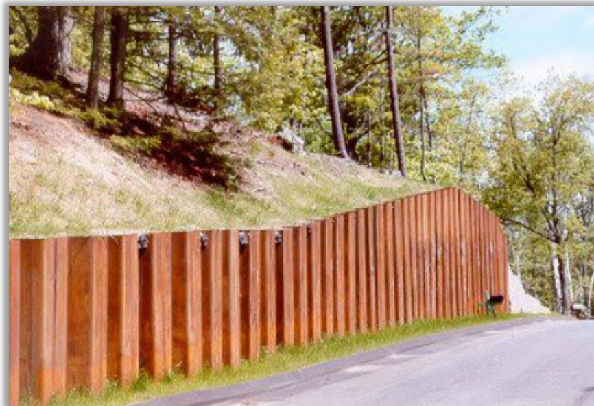
Figure 8: Sheet piling wall
