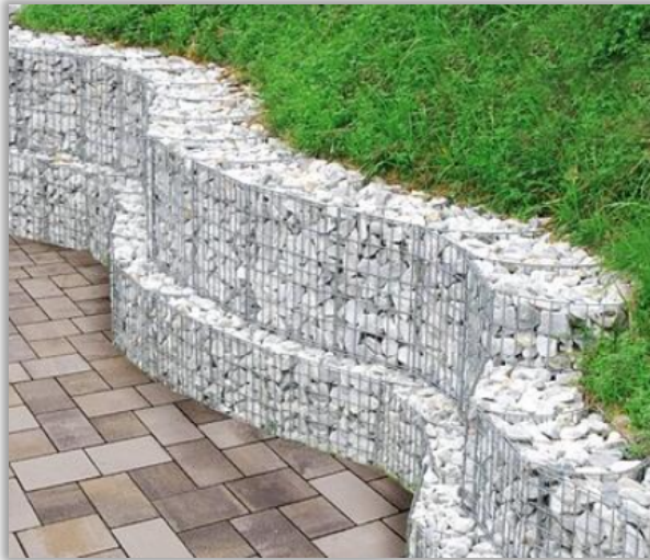
Figure 4: Gabion Walls
