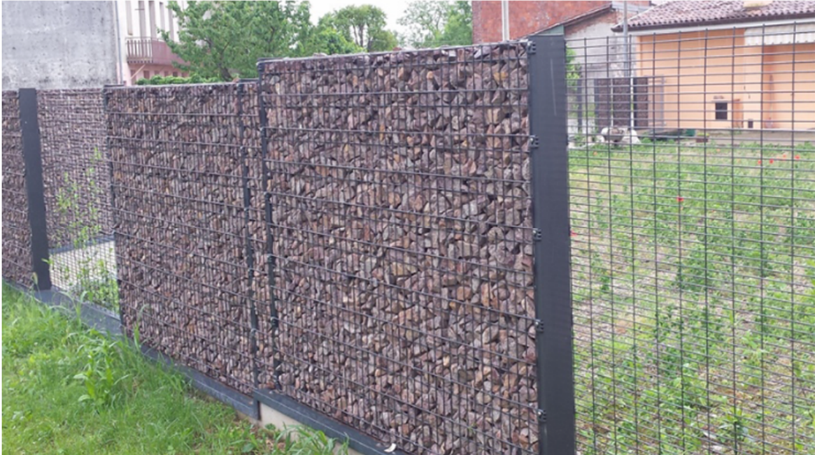
Figure 12: Gabion free standing wall
