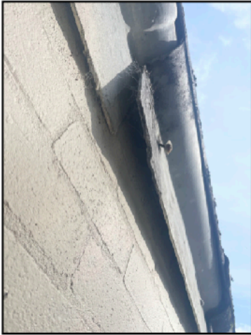
Raised Timber Fasciae on the Lean-to Structure
