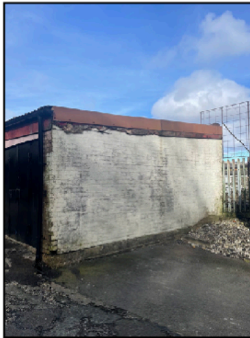
South Eastern Elevation of the Garage Block
