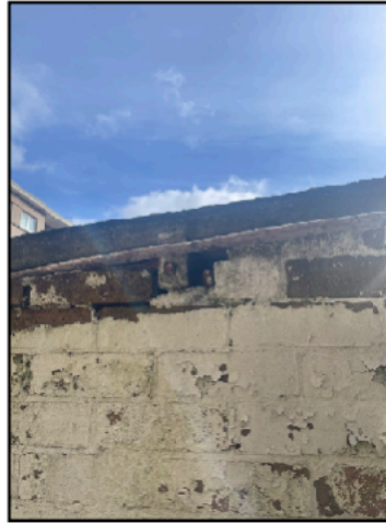
Apertures in the Brickwork on the Lean-to Structure
