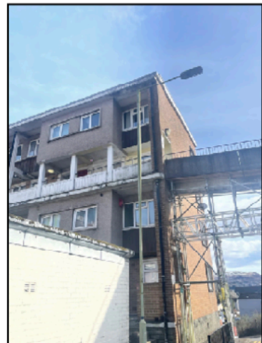
South Eastern Elevation of the Main Building
