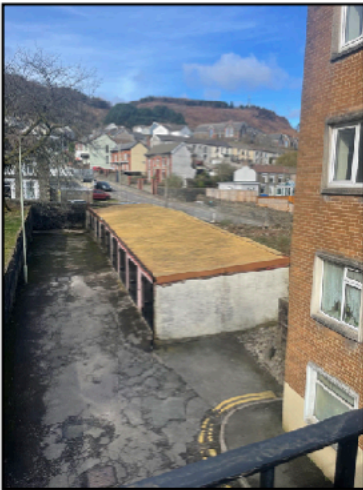
Garage Block to the North West of the Main Building
