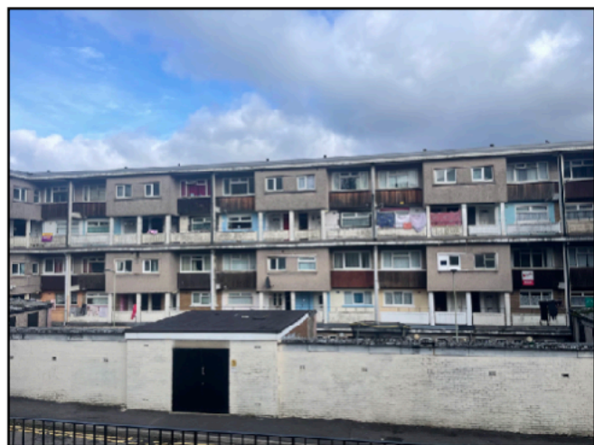
Western Elevation of the Main Building
