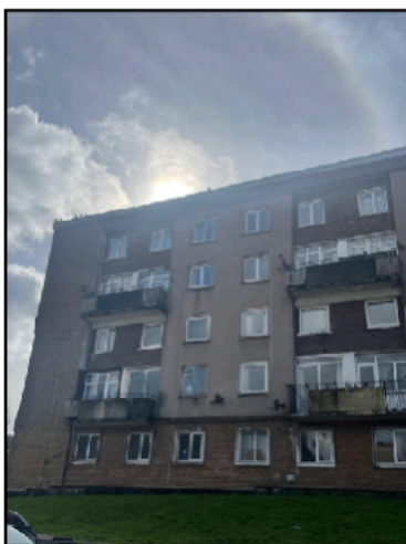
Eastern Elevation of the Main Building
