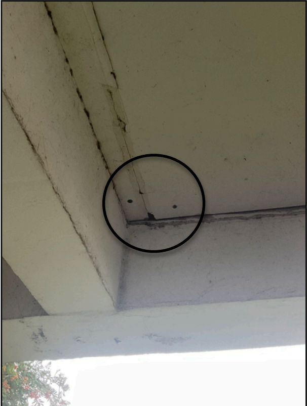
Small Aperture within the Ceiling of the Undercroft Car Parking Area
