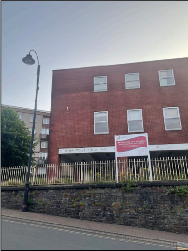
Eastern Elevation of the Main Building
