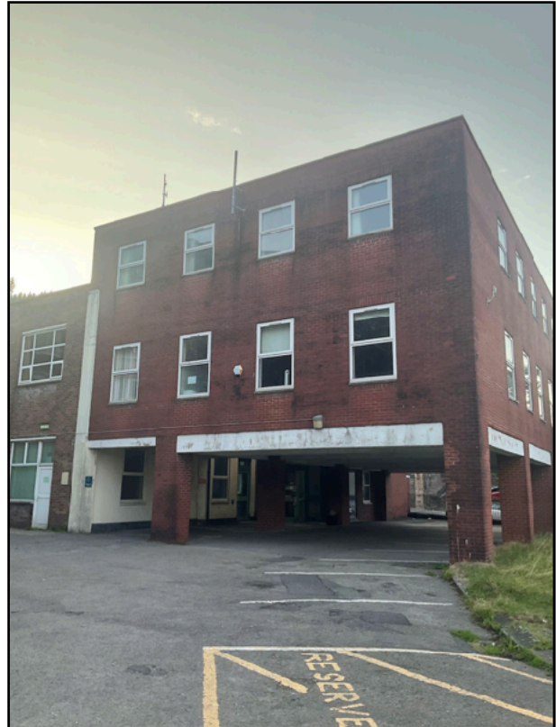
Southern Elevation of the Main Building with Undercroft Car Parking Area
