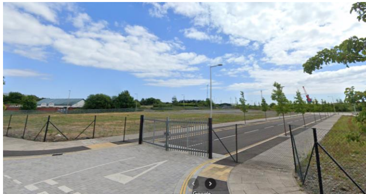
Figure 2: View from the north looking south along the recently constructed road and towards plot E7/E8 and ABP land further south
