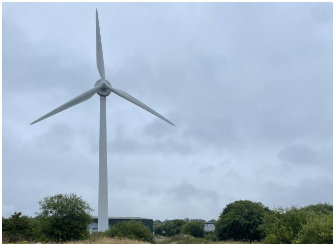
Existing Structures located within close proximity to the application site
