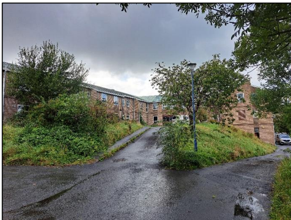
Figure 6. Main Building and Road
