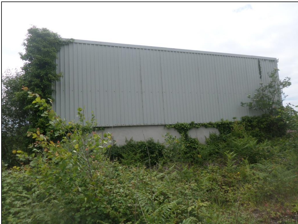
Photo 8: Northern elevation of prefabricated building (view looking south).
