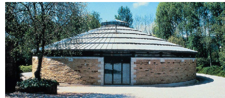
David Mellor Factory Roof (Standing Seam Metal Roof)
