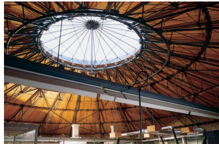
David Mellor Factory Skylight /Ceiling
