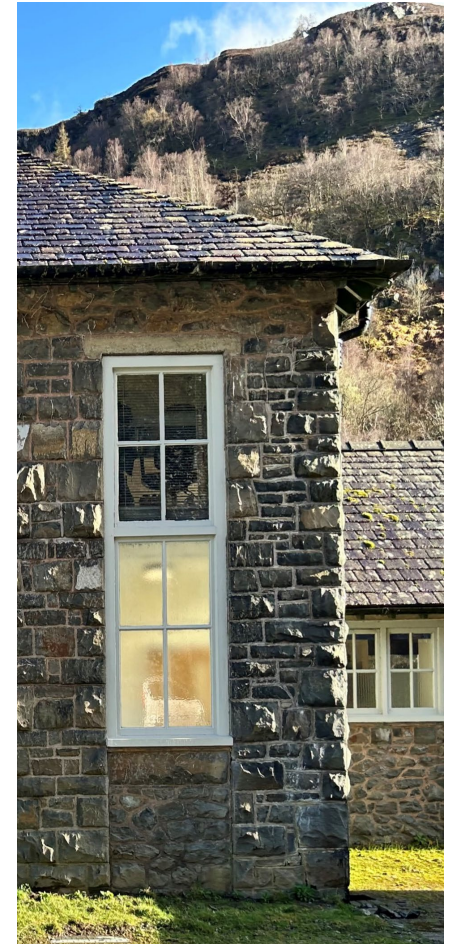
Existing Stone/Window Detailing
