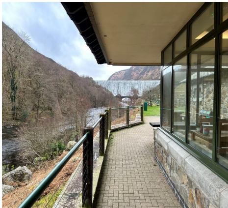
Existing Restaurant Windows, Low Wall/Sill and Eaves Overhangs
