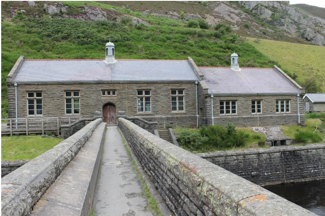
Image EDP A1.9: View from the bridge of the northernmost power station building illustrating its appearance.
