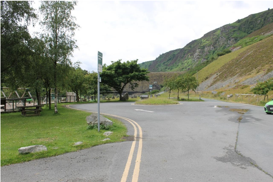
Image EDP A1.5: View towards Caban Coch Dam from the western part of the site illustrating how an appreciation of the dam is obscured by intervening trees and play equipment and how the vehicle turning circle is a prominent modern feature of the space.
