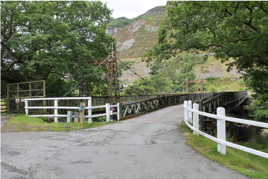
Image EDP A1.13: View from the east illustrating the appearance of the two bridges that provide access to Elan Village at the western edge of the conservation area.
