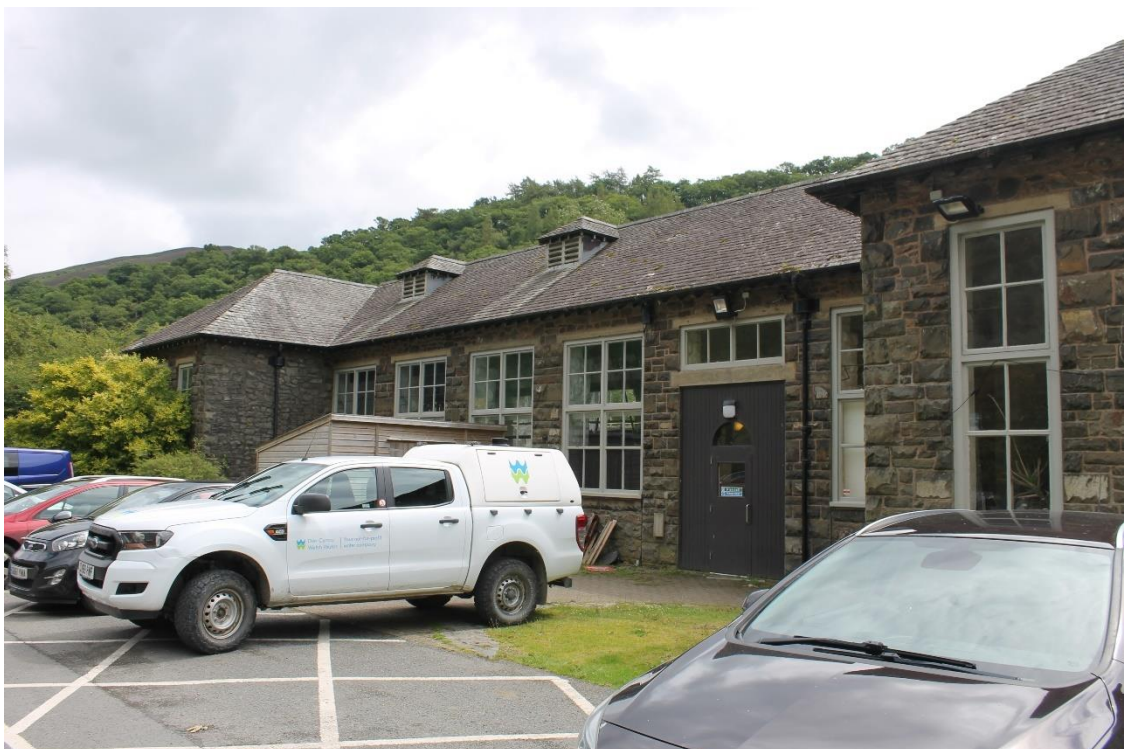
Image EDP A1.22: View of part of the north elevation of the Visitor Centre building illustrating the fenestration and modern inserted door.
