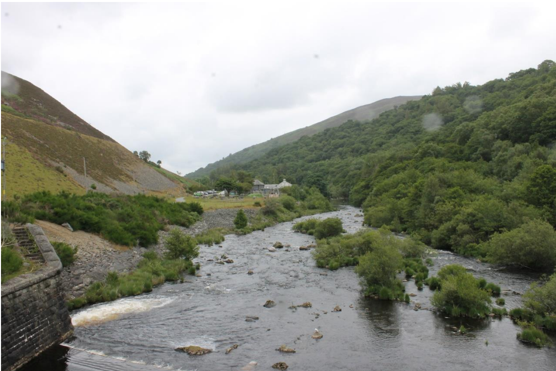
Image EDP A1.12: View towards the Visitor Centre building from the bridge between the power station buildings. This view illustrates how the material finish of the building accords with that of the listed elements and also how the modern features set around the Visitor Centre building are also prominent elements of the view.
