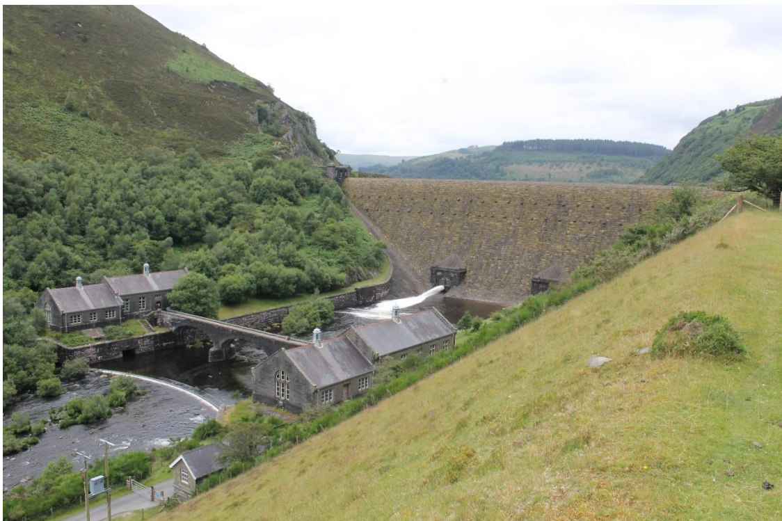
Image EDP A1.10: View from the top of the spoil tip to the north-east illustrating the close association between the power station buildings, the bridge and the Caban Coch Dam
