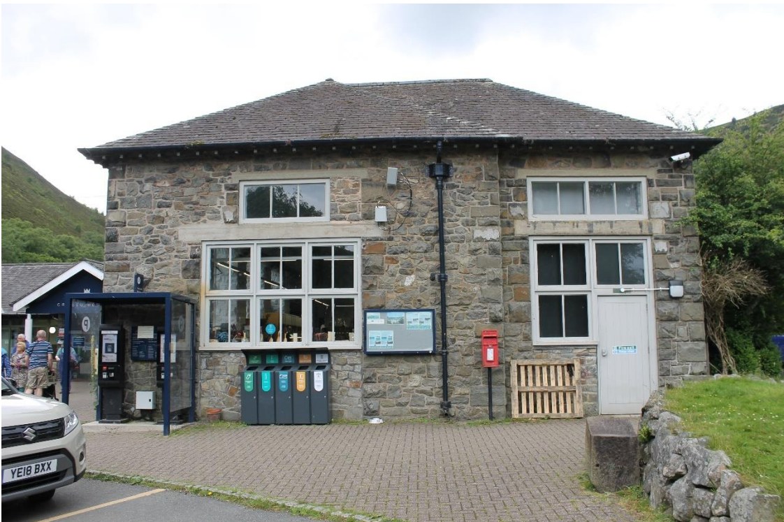
Image EDP A1.20: View of the eastern elevation of the Visitor Centre building showing where two original large entrances were located.
