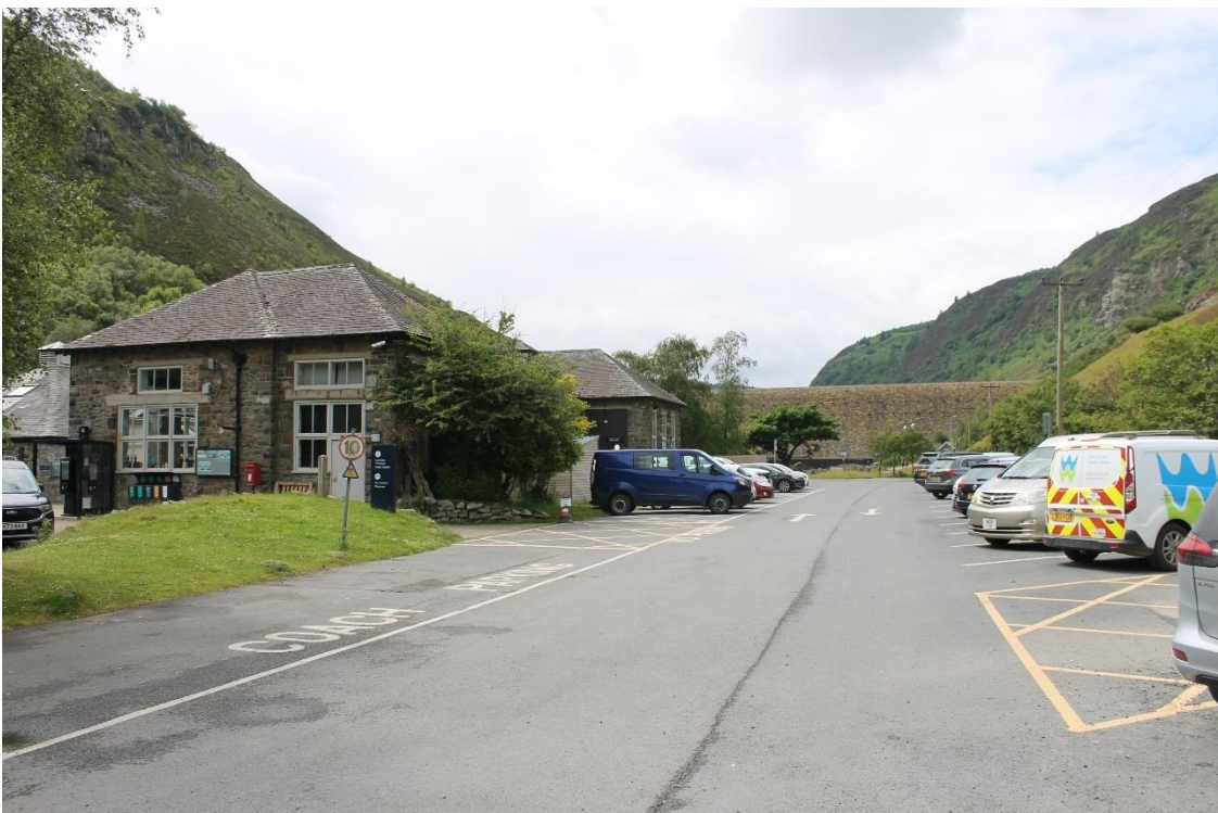
Image EDP A1.4: View towards Caban Coch Dam from c.400m to the east illustrating how it can be seen above intervening features due to its large size.
