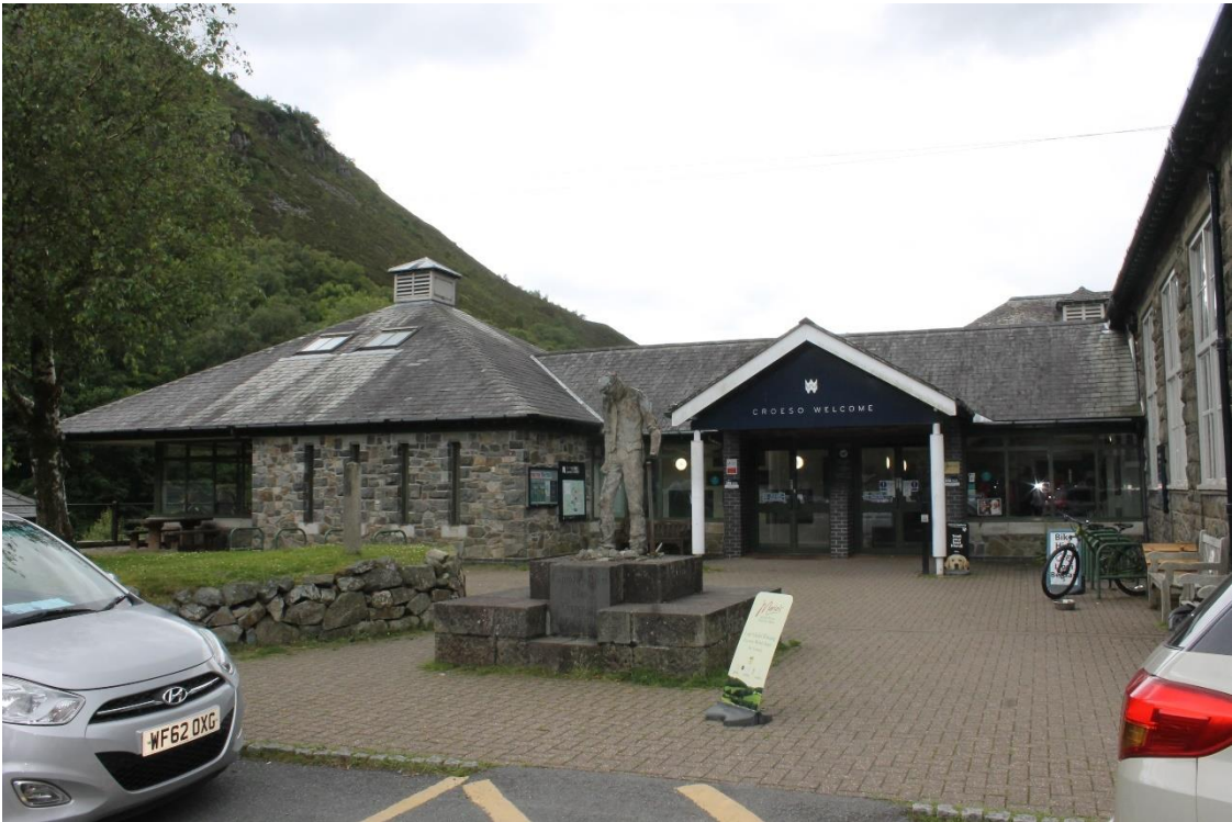
Image EDP A1.25: View of the eastern end of the Visitor Centre building, illustrating the frontage of the modern entrance hall and restaurant extension of the 1980s.
