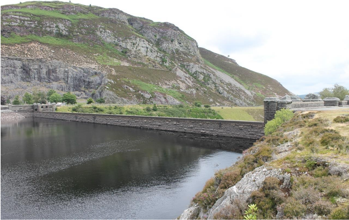
Image EDP A1.1: View of Caban Coch Dam from the south-west and illustrating its appearance from the reservoir.
