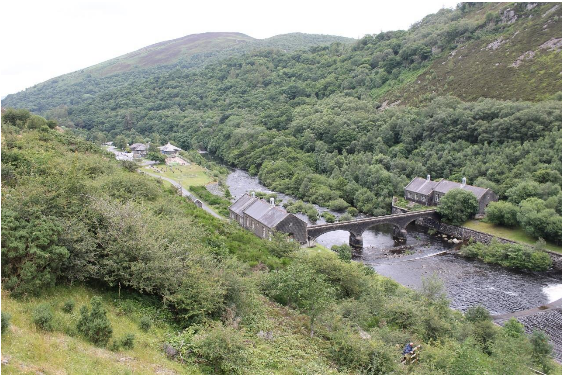
Image EDP A1.3: View to the east along the Elan Valley from the northern tower of the Caban Coch Dam. The view shows the hydro-electric power station buildings and bridge with the Visitor Centre building and its related infrastructure beyond. The similar use of materials between the buildings can be seen as can the contrast between the well-preserved historic buildings in the foreground and the modern development around the Visitor centre.
