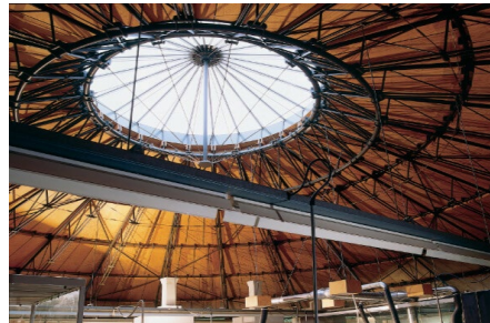
David Mellor Factory Skylight /Ceiling
