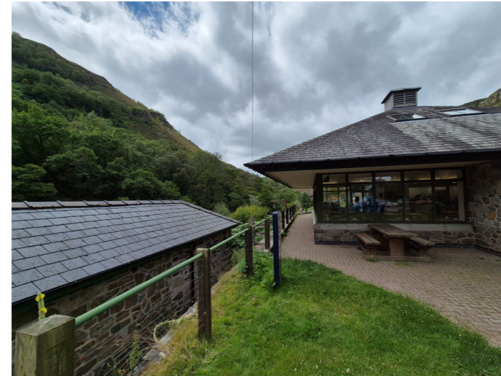
Accessibility and wayfinding on river side toward the dam to be improved
