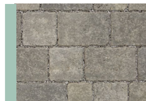
Permeable block paving Location: carpark space
