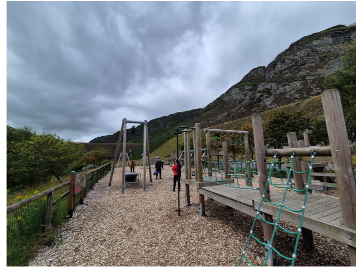
Dam view obstructed with existing play area
