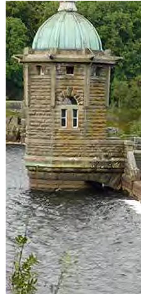
Elan Valley Dams Kiosk Roof (Standing Seam Patinated Metal Roof)
