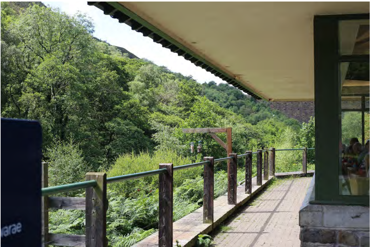
Photo 3: View from existing decking overlooking Afon Elan.
