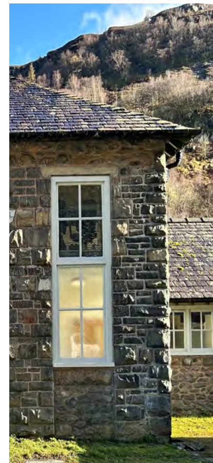
Existing Stone/Window Detailing
