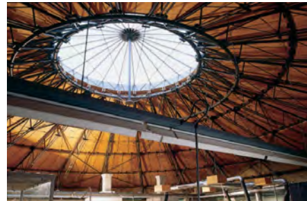
David Mellor Factory Skylight /Ceiling
