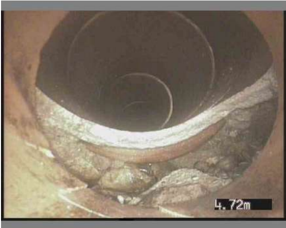
4-1-8A, 00:00:59, 4.72 m Survey abandoned, UNABLE TO PASS
