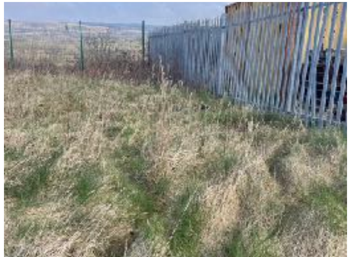
10. Northeast corner of site. Metal fencing to east and green fencing to north.
