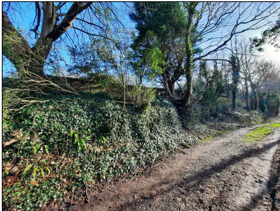
Plate 12: Downslope to Track to South-west (Alongside Stockpile)
