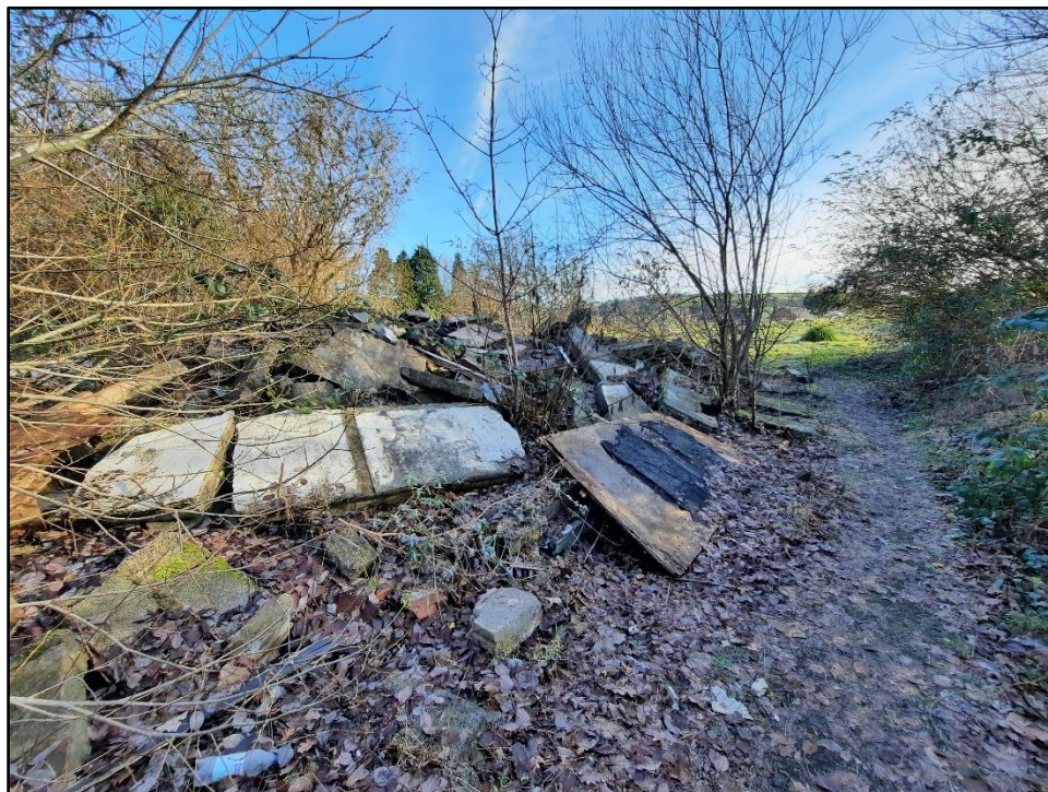
Plate 4: Stockpile of Demolition Rubble (eastern margins) Narrow path through to main part of site on right.
