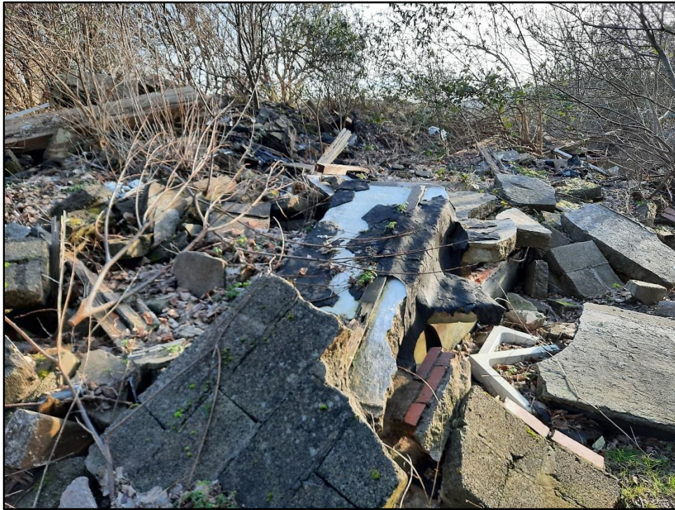
Plate 3: Stockpile of Demolition Rubble (north-western margins)
