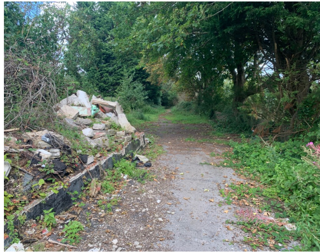
Former road that led to Tudor Inn.
